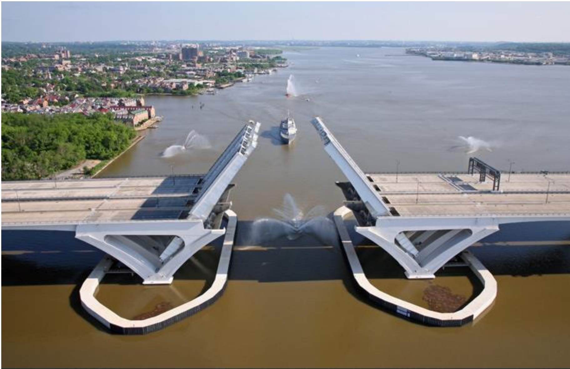
CSA PROPOSAL - Bascule draw span similar to this new Woodrow Wilson I-95 Bridge near Washington DC
