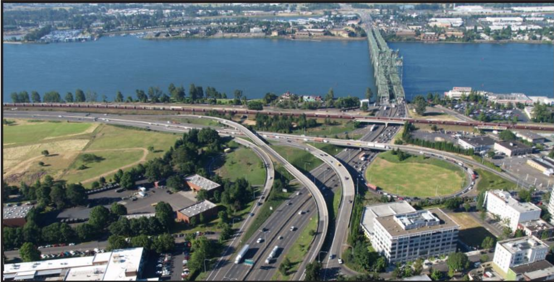
Looking South from Vancouver
