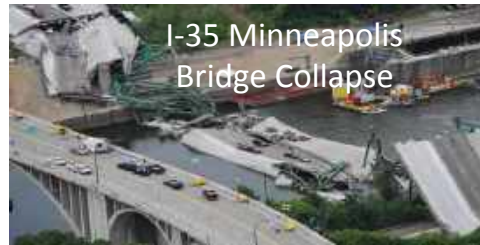
250 tons- asymmetrical loading
